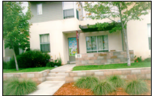
Low retaining walls in the front yard
